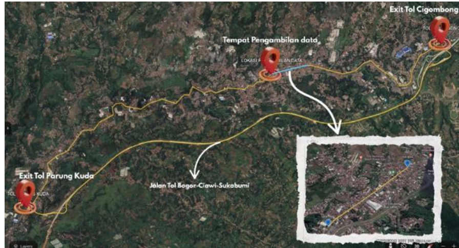
Figure 1 Siliwangi Cicurug-Benda Road segment, located between STA 30+000 and STA 31+000 (source: google maps)
